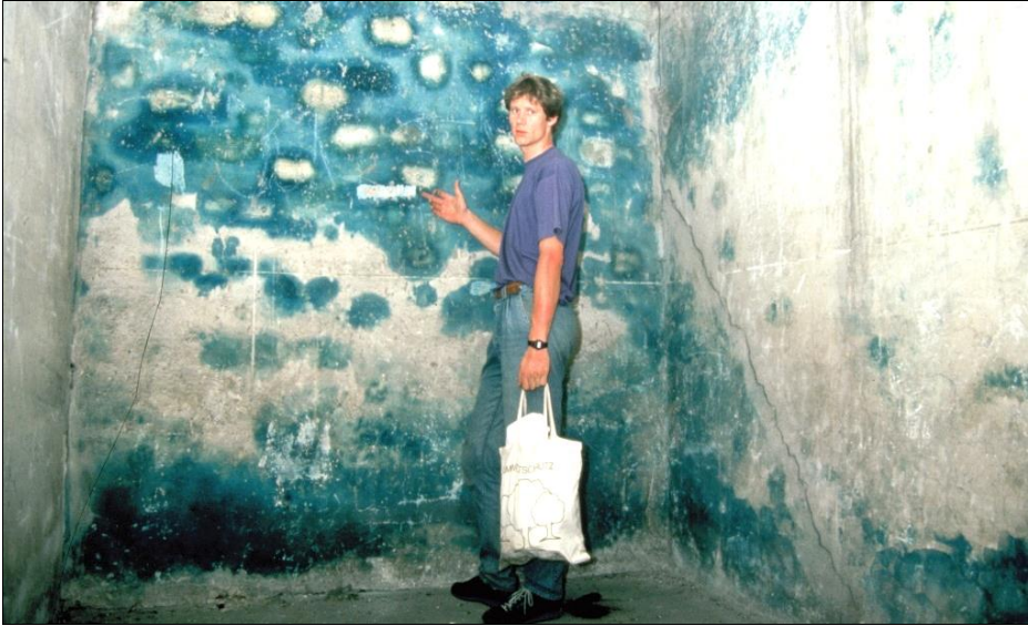
Illustration 19: The 26-year-old Geremar Rudolf inspects a Birkenau delousing chamber (building no. BW 5a) for sampling. Its wall has an intensive blue hue.
