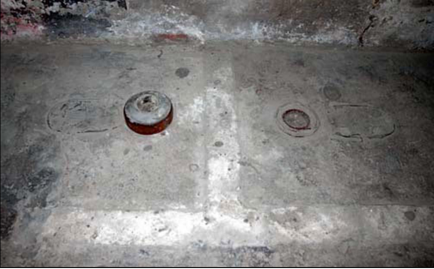
Illustration 6: Two toilet drains with imprints of the toilets and the stall walls still visible on the floor of what tourists experience as “the gas chamber” at the Auschwitz Main Camp. The toilets were added in 1944 in the wash room adjoining the morgue (aka “gas chambers”) when the building was converted to an air-raid shelter, and accidentally included in the “gas chamber” when the shelter’s partition walls were torn down by the Auschwitz Museum in 1947 during their “reconstruction.”
