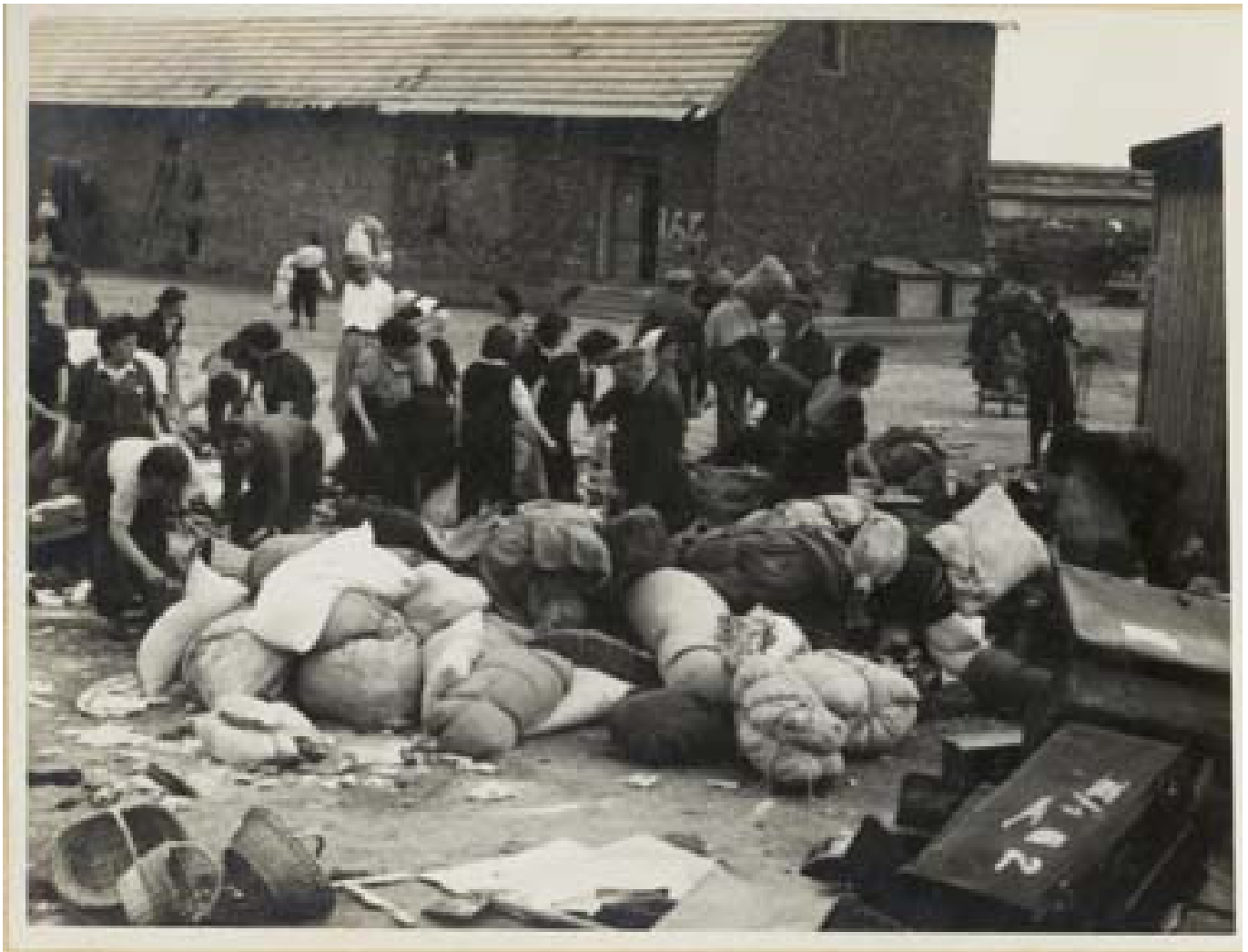
Possibly loading of the fabrics onto racks for treatment. The loads seem to be carried to the treatment building (?) at top left. A loaded rack seems to be visible to the right on the roadway.
